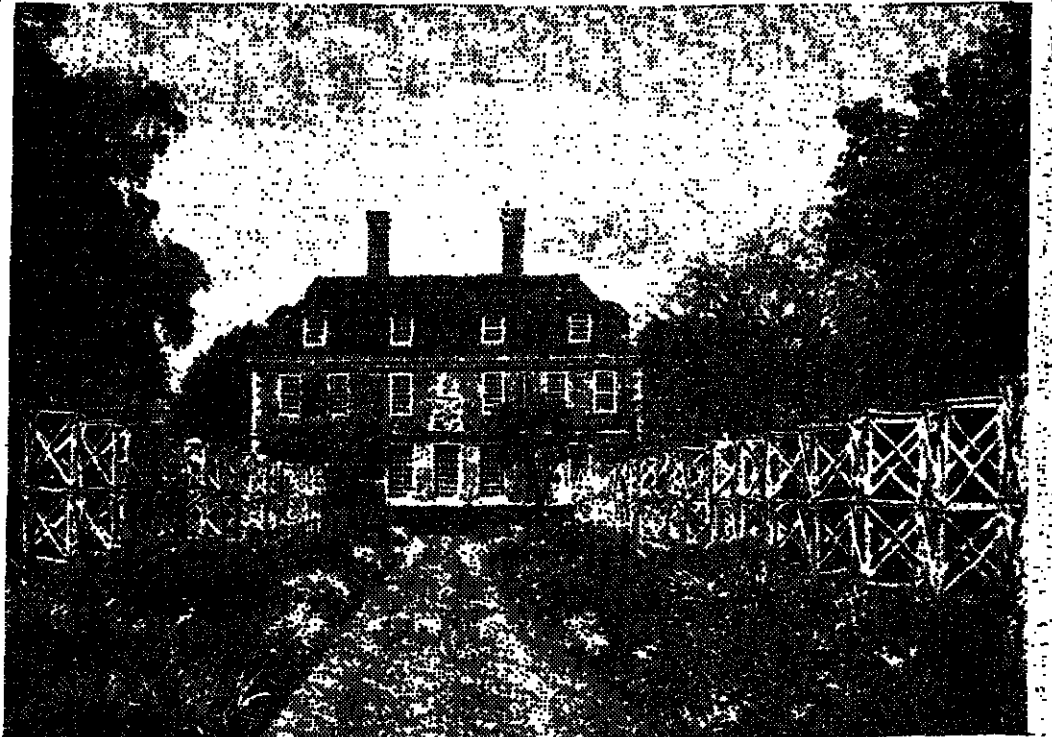
The Salutation, Sandwich, Kent where the Jekyll garden and Lutyens house are being carefully restored and opened occasionally to the public.
